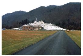
Figure 2b. The 300' Green Bank telescope after November 15, 1988, 9:43 pm. Image courtesy of NRAO/AUI.
